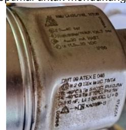
GAMBAR 2.2 *NAMEPLATE PRESSURE TRANSMITTER* ENDRESS HAUSER
